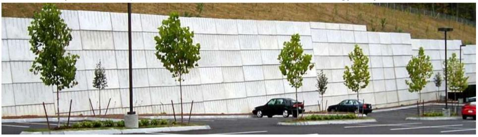
Typical EVERWALL application: a gravity retaining wall to support a hillside and expand a needed parking area.
