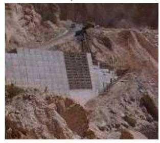
50 feet high EVERWALL gravity wall nearing completion in Yemen.
