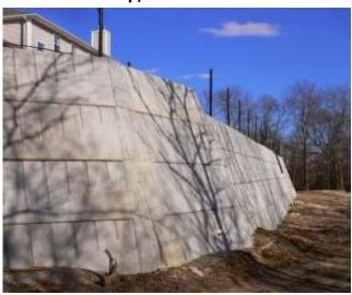
EVERWALL replacement, for a failed segmental block retaining wall, Long Island, NY, USA
